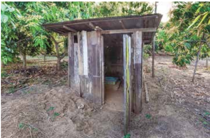
Typical Pit Latrine.
